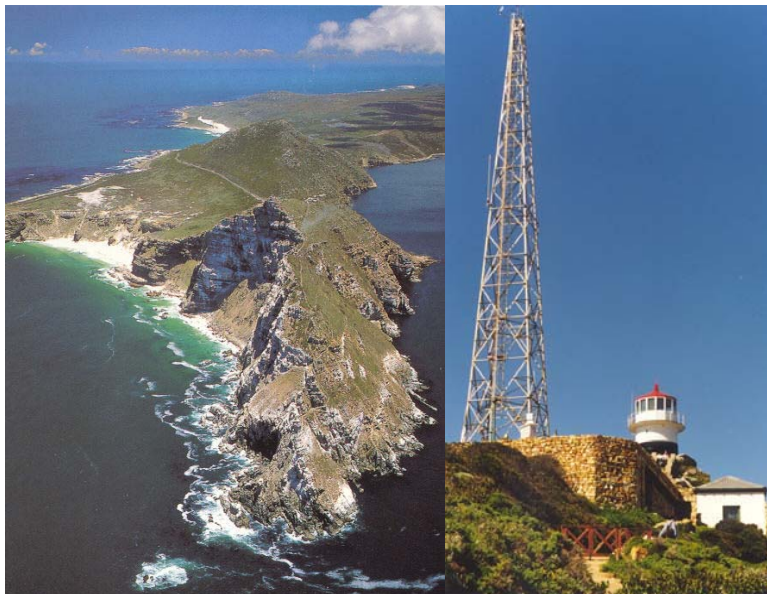
Figure 1: Aerial view of Cape Point and photo showing the air intake mast together with the laboratory building, which is partly integrated into the surrounding rock face.
