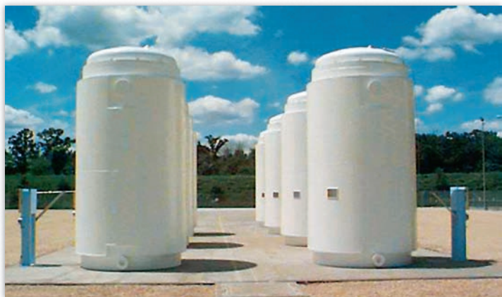
▲ FIGURE 13.17 Spent fuel is being stored temporarily in large, aboveground “dry casks” at many nuclear power plants.
