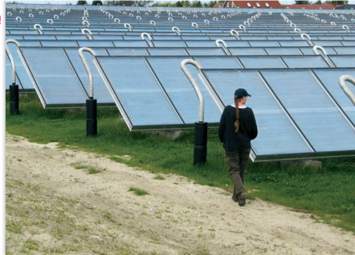
▲ FIGURE 13.29 Solar water heaters can be scaled up to provide hot water and space heating for whole cities.
