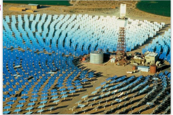
▲ FIGURE 13.30 A "Power Tower" is a form of concentrated solar thermal electrical generation. Thousands of movable mirrors focus intense energy on the tower, where fluid is heated to drive a steam turbine.
