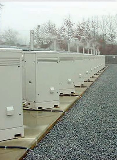
◀ FIGURE 13.37 The Long Island Power Authority has installed 75 stationary fuel cells to provide reliable backup power.
