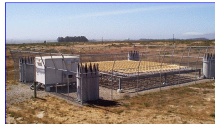
Typical NPN Profiler Site Equipped With RASS. (Use mouse to identify specific components.)
