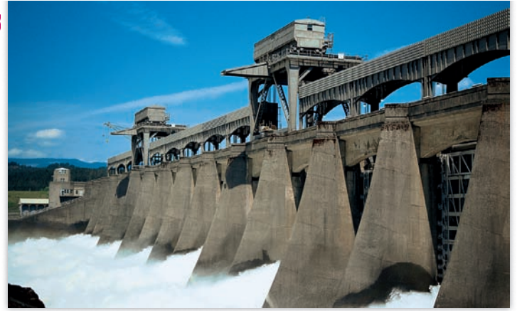
▲ FIGURE 16.5 Every major federal project in the United States must be preceded by an Environmental Impact Statement.
