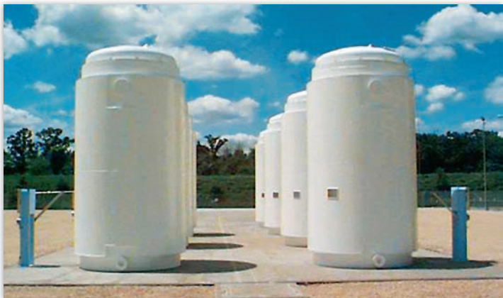
▲ FIGURE 13.17 Spent fuel is being stored temporarily in large, aboveground “dry casks” at many nuclear power plants.
