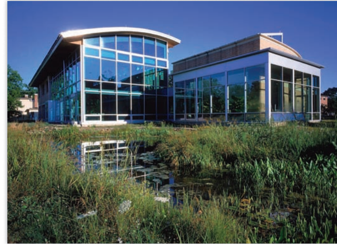
▲ FIGURE 16.18 The Adam Joseph Lewis Center for Environmental Studies at Oberlin College is designed to be self-sustaining even in northern Ohio's cool, cloudy climate. Large, south-facing windows let in sunlight, while 370 m 2 of solar panels on the roof generate electricity. Natural wastewater treatment, including a constructed wetland, purifies wastewater.
