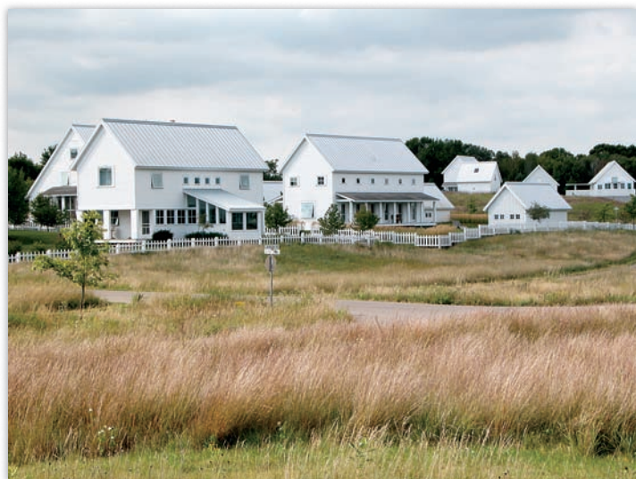
▲ FIGURE 15.14 Jackson Meadows, an award-winning cluster development near Stillwater, Minnesota, groups houses at sociable distances and preserves surrounding open space for walking, gardening, and scenic views from all houses.
