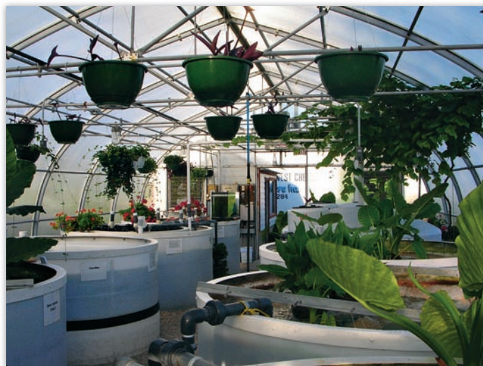
▲ FIGURE 11.30 This Wisconsin cheese factory treats its effluent by passing it through a series of large tanks in which plants, bacteria, algae, and other aquatic organisms filter the water and remove organic material, suspended solids, and nutrients.
