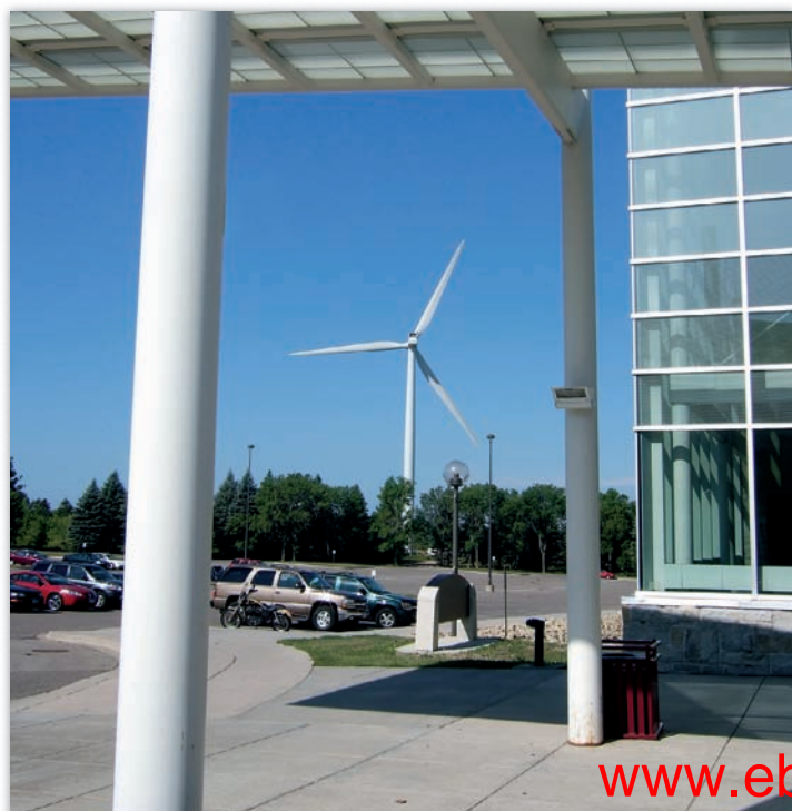
▼ FIGURE 16.19 Many schools have installed their own wind turbines. Although a large turbine may cost about $2 million, the payback can be as short as ten years.
