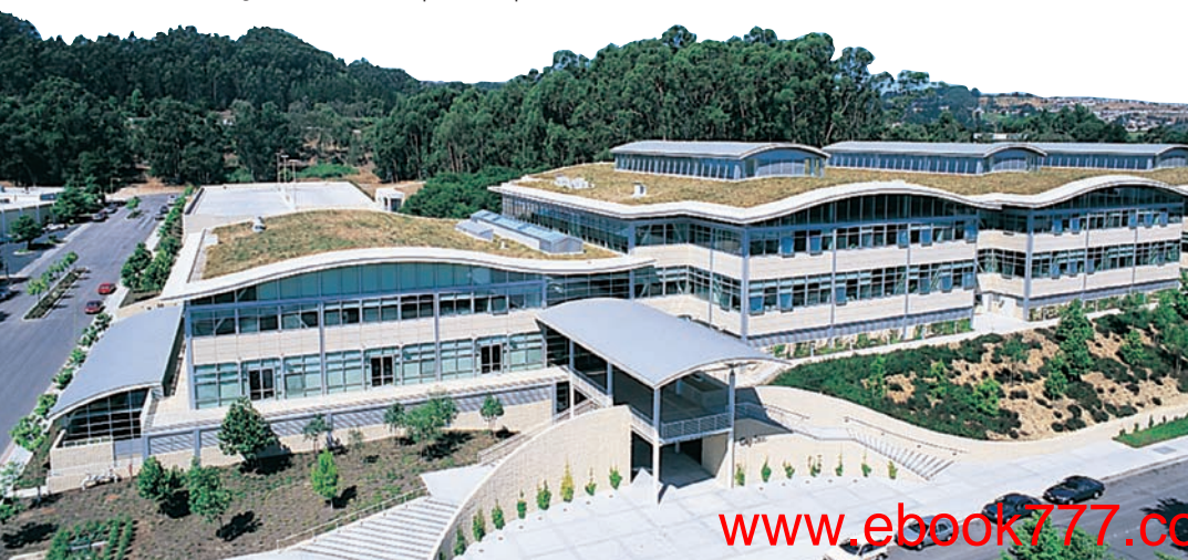
▼ FIGURE 15.24 The award-winning Gap, Inc. corporate offices in San Bruno, California, demonstrate some of the best features of environmental design. A roof covered with native grasses provides insulation and reduces runoff. Natural lighting, an open design, and careful relation to its surroundings all make this a pleasant place to work.
