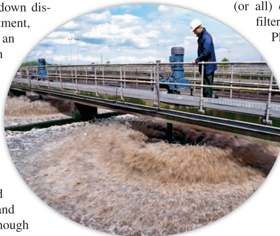
◀ FIGURE 11.28 In conventional sewage treatment, aerobic bacteria digest organic materials in high-pressure aeration tanks. This is described as secondary treatment.
