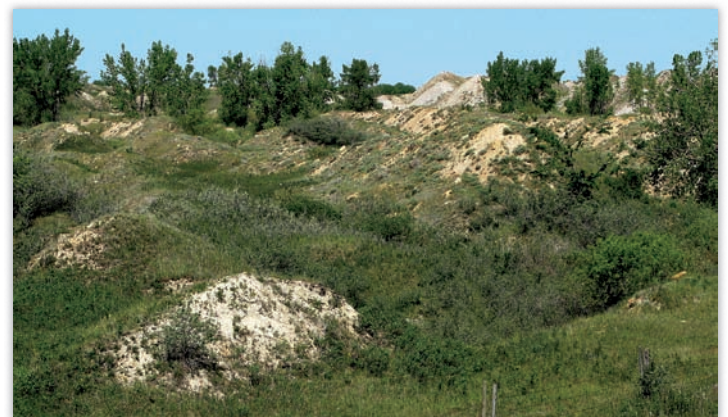
▲ FIGURE 12.14 This surface coal mine in Saskatchewan was abandoned a century ago. Plants are slowly vegetating the waste rock piles, but the land has little economic or biological value.
