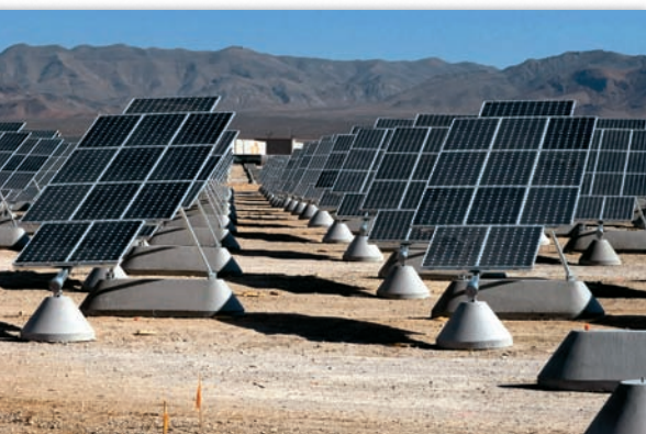
(a) Base-load power facility
