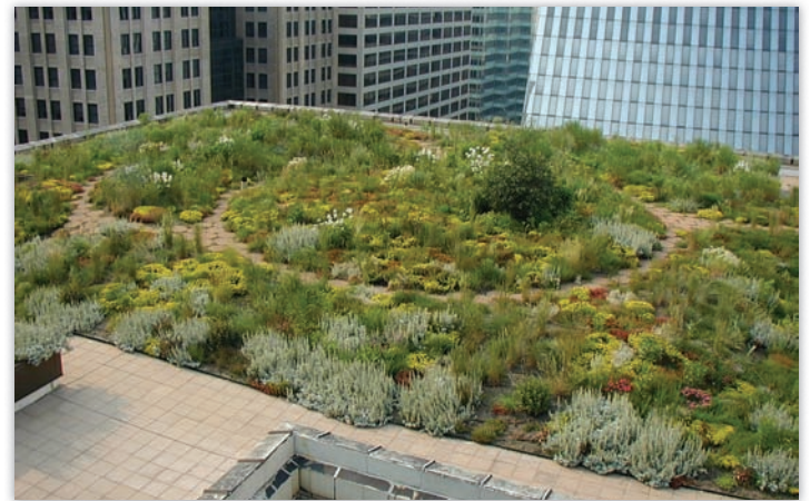
▲ FIGURE 15.13 This award-winning green roof on the Chicago City Hall is functional as well as beautiful. It reduces rain runoff by about 50 percent, and keeps the surface as much as 30°F cooler than a conventional roof on hot summer days.
