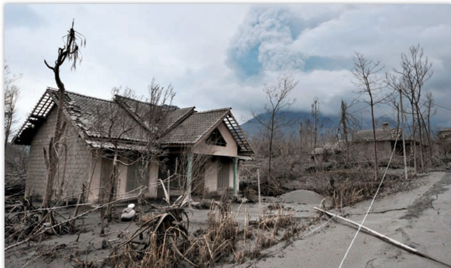
▲ FIGURE 12.18 Volcanic ash covers damaged houses and dead vegetation after the November 2010 eruption of Mt. Merapi (background) in central Java. More than 300,000 residents were displaced and at least 325 were killed by this multiday eruption.
