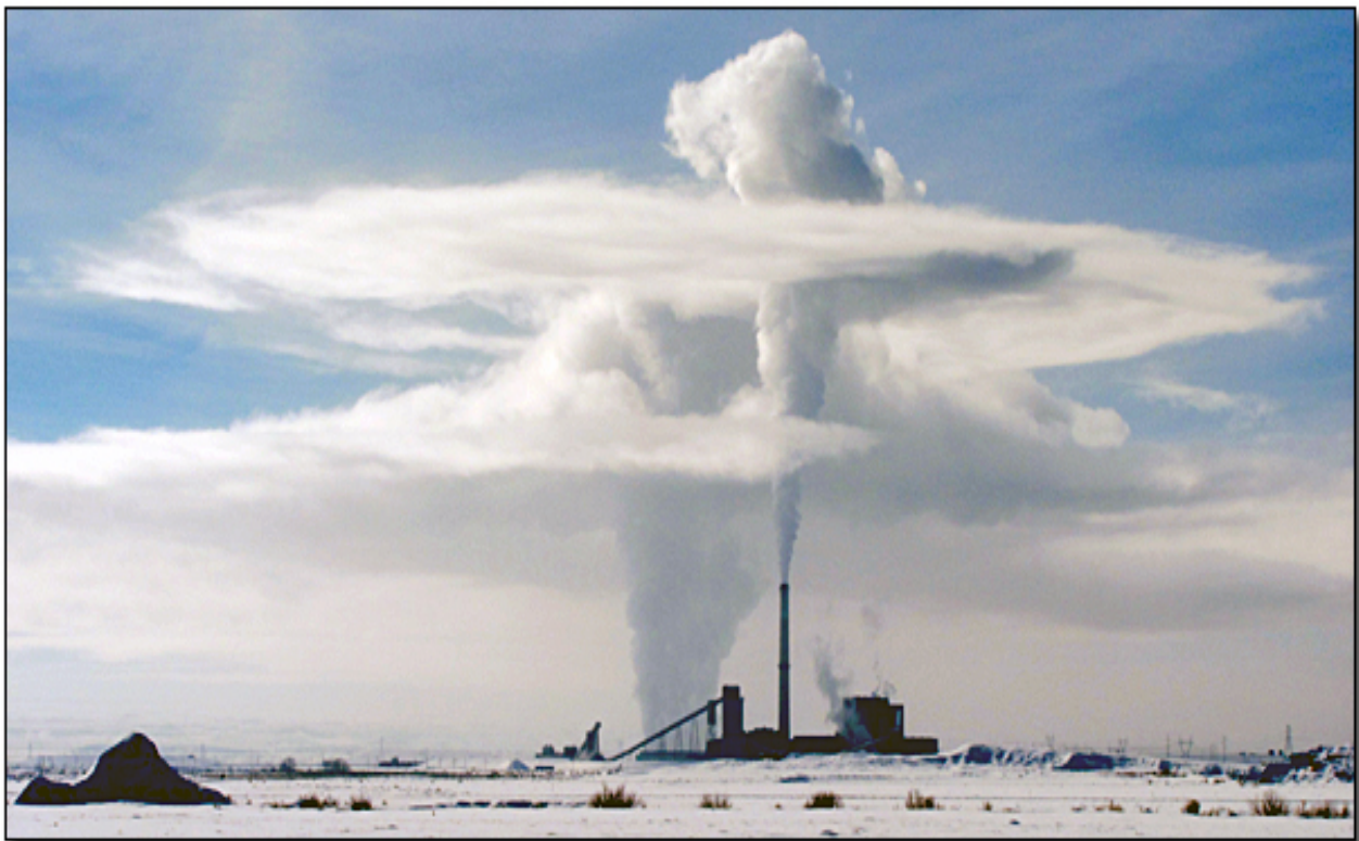
Figure 8-42. Bonanza power plant with buoyant exhaust plume and water vapor from the cooling ponds. The top of the stack is 1715.8 m and the plume generally rose an additional 2 to 3 stack heights before leveling out in the 1900 to 2200 m range. In the winter of 2013 the inversion top was generally between 1600 and 1750 m.
